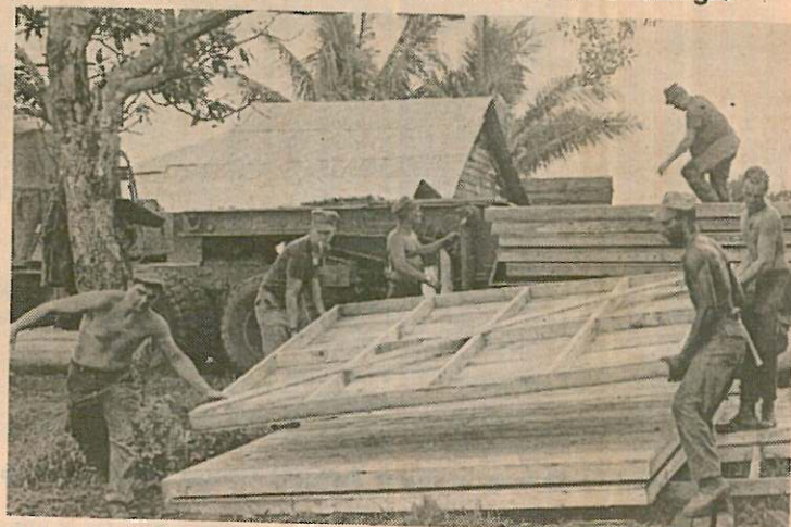
Unloading prefabricated floors are Navymen of Battalion 58.
