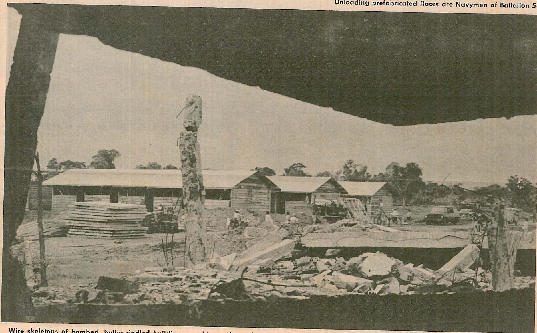
Wire skeletons of bombed, bullet-riddled buildings provides a dramatic contrast to the nearly completed buildings having the finishing touches put on.
